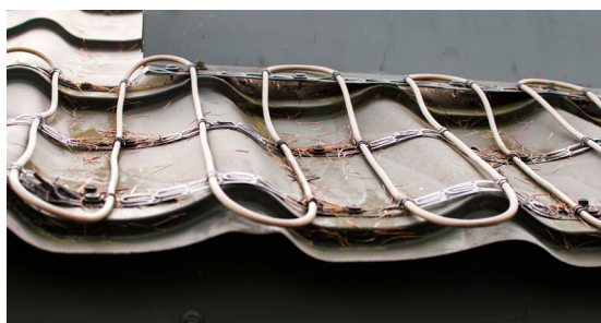
34000003 - screwed onto roof surface
